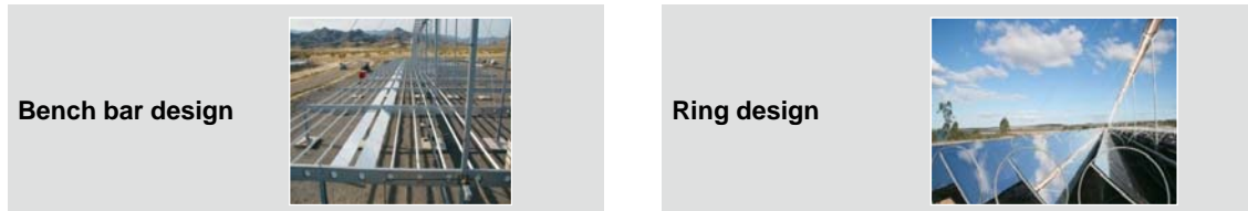
Figure 20: Linear Fresnel support structure designs
