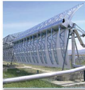
Torque tube with cantilever arms
