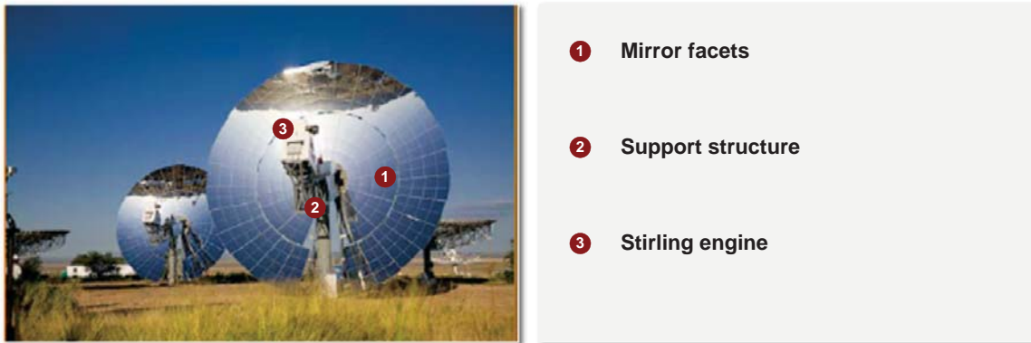
Figure 18: Components of a dish Stirling system
