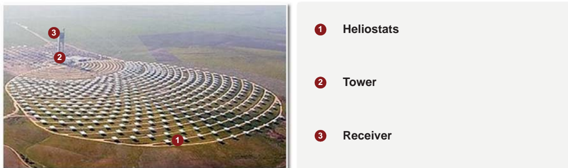
Figure 17: Components of a solar tower field
