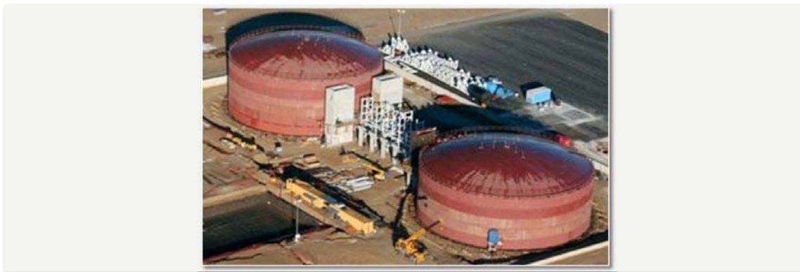
Figure 21: The two-tank storage system
