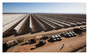
Phase one of Morocco's vast \$9bn Ouarzazate solar power plant provides 160MW of its ultimate 580MW capacity. Photograph: Graeme Robertson for the Guardian
