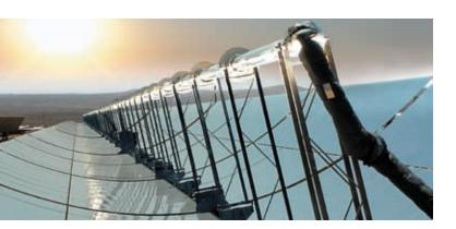
Parabolic Trough plants use line-concentrating parabolic trough collectors which reflect the solar radiation into an absorber tube. Synthetic oil circulates through the tubes and is heated up to approximately 400°C.
