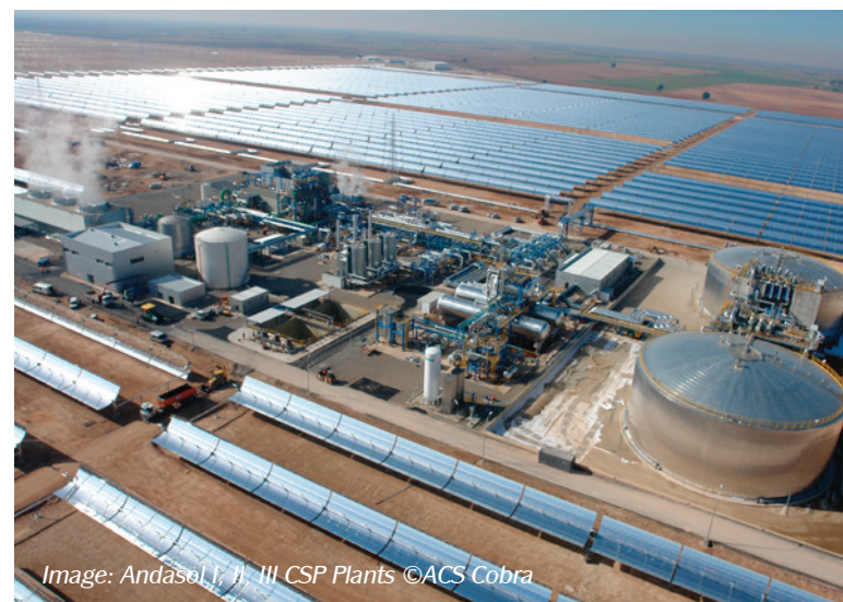
Figure 5: Parabolic trough plant with thermal storage
