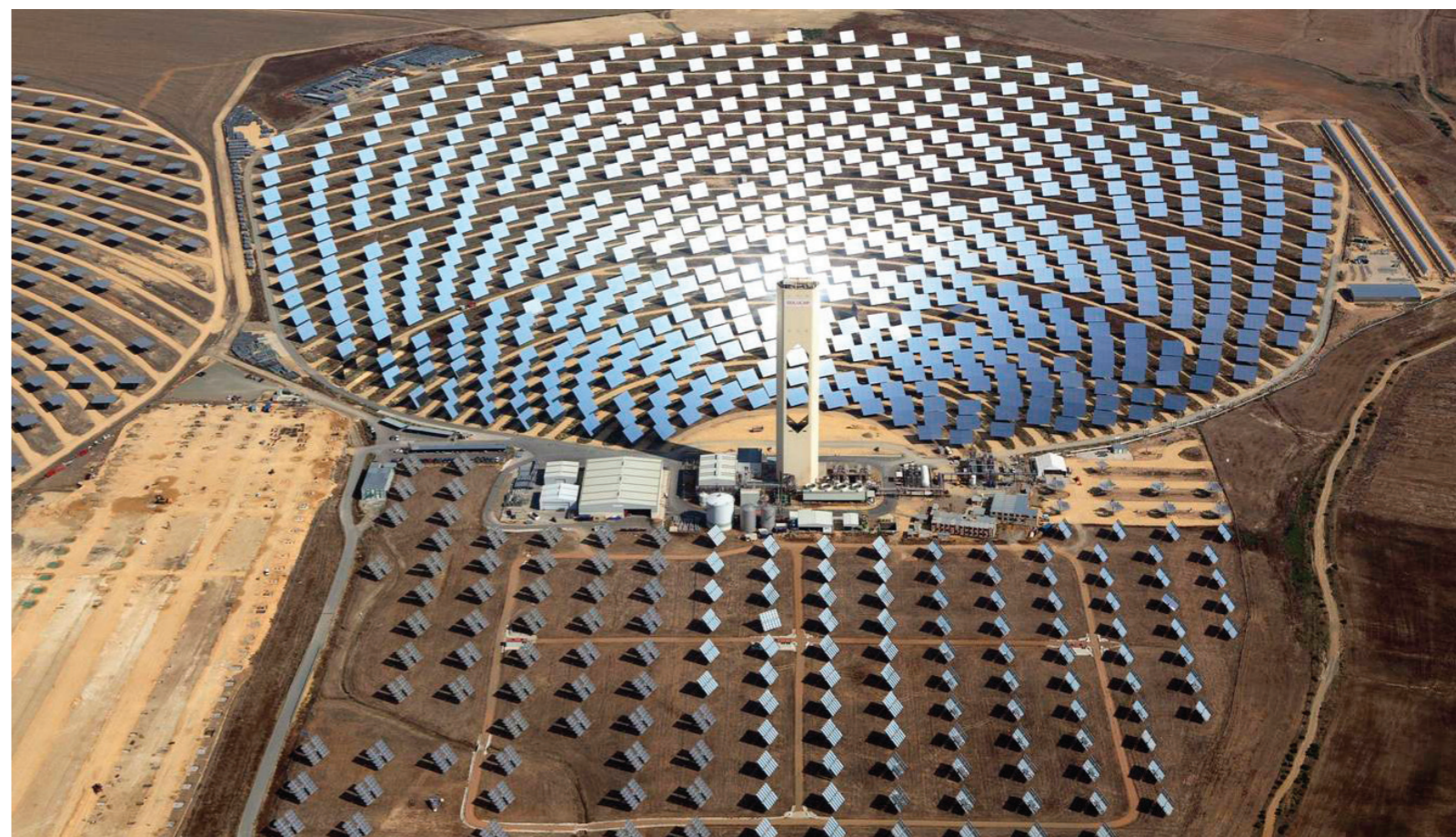
Image: 10 MW STE plant co-located with 1 MW PV in the Solucar complex, Seville, Spain ©Abengoa Solar
